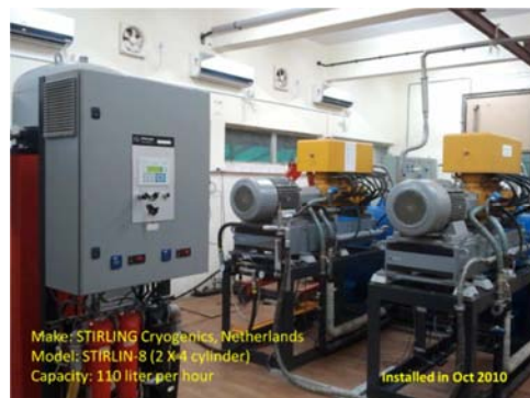
Figure 1. STIRLIN-8 Liquid nitrogen plant at LTF.
