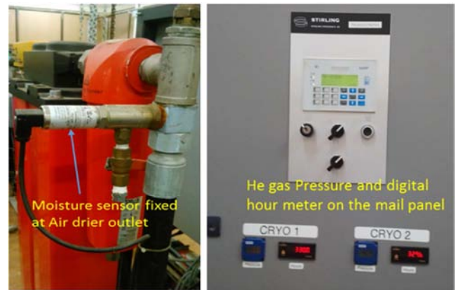
Figure 4. Modification of the STIRLIN8 plant.
