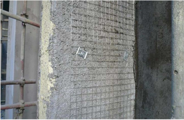
Figure 9. Rigid polyurethane foam composite polystyrene particle insulation slurry wall.
