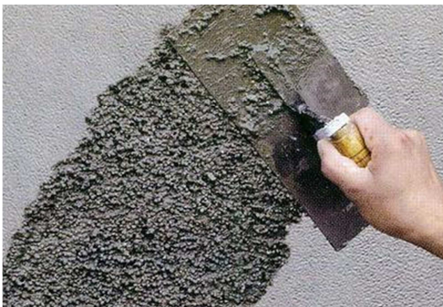
Figure 6. Polystyrene Granule Insulating Slurry.
