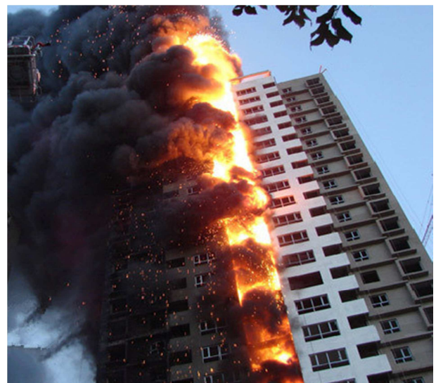
Figure 11. Exterior insulation material cause fire.
