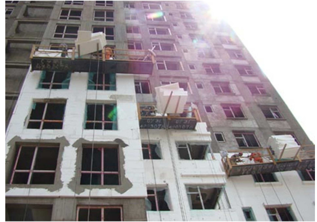
Figure 3. Construction of polystyrene (EPS) board.
