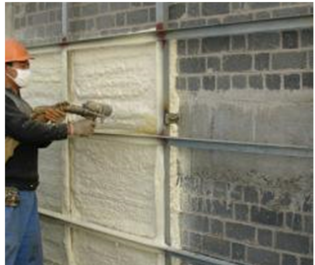
Figure 7. Spraying polyurethane rigid foam.
