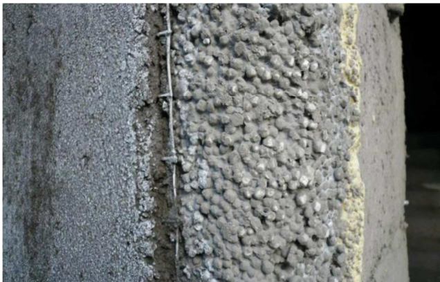
Figure 5. Rigid polyurethane foam and Polystyrene Granule Insulating Slurry.
