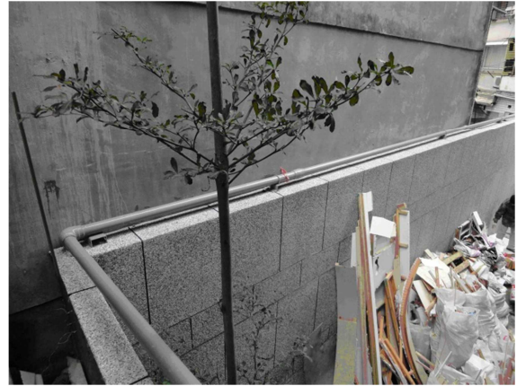
Figure 7. Open-Air Gas Steel Pipes on the Top of the New North Wall.
