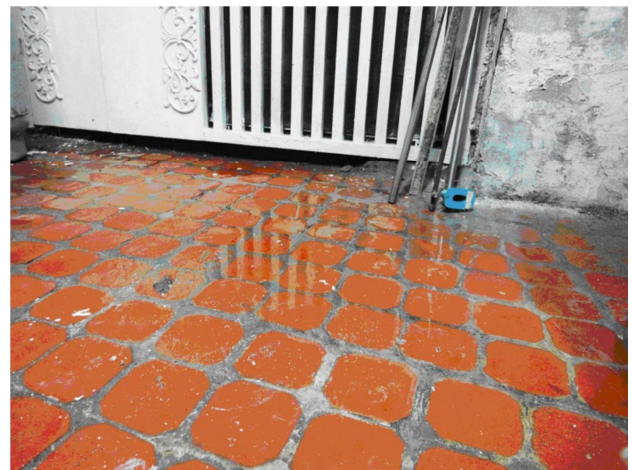
Figure 6. Leakage on the Plaintiff's Kitchen Floor.
