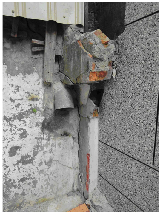
Figure 5. Cracks on the Plaintiff's Kitchen outside Wall.
