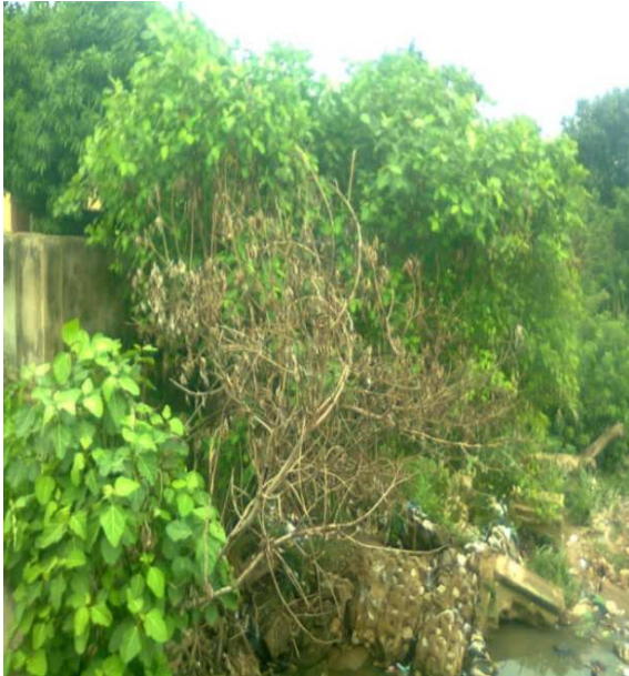
Plate 1. Building's fence in the river at phase 3
