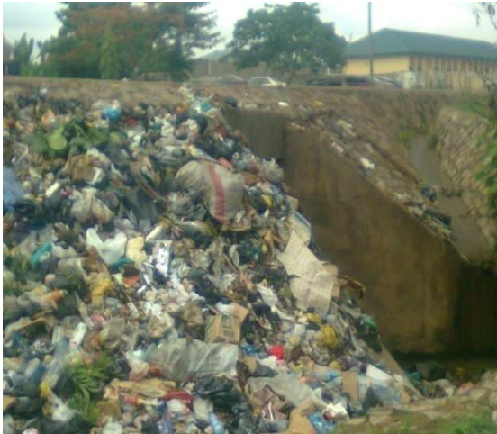
Plate 3. Debris by the bridge edge along phase 3.
