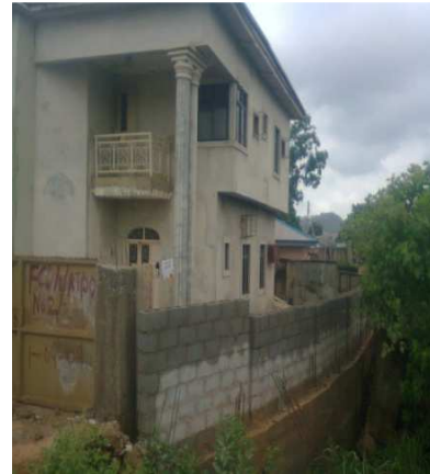
Plate 2. House encroaching on the river at phase 2
