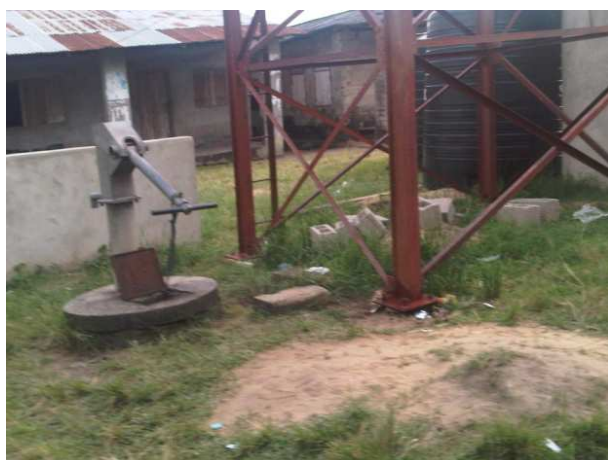
Figure 2. An abandoned hand pump fitted borehole at Ibeshe.
