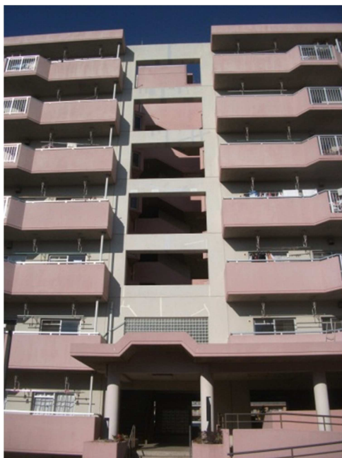
Figure 15. Front View of Reinforced Concrete Housing.
